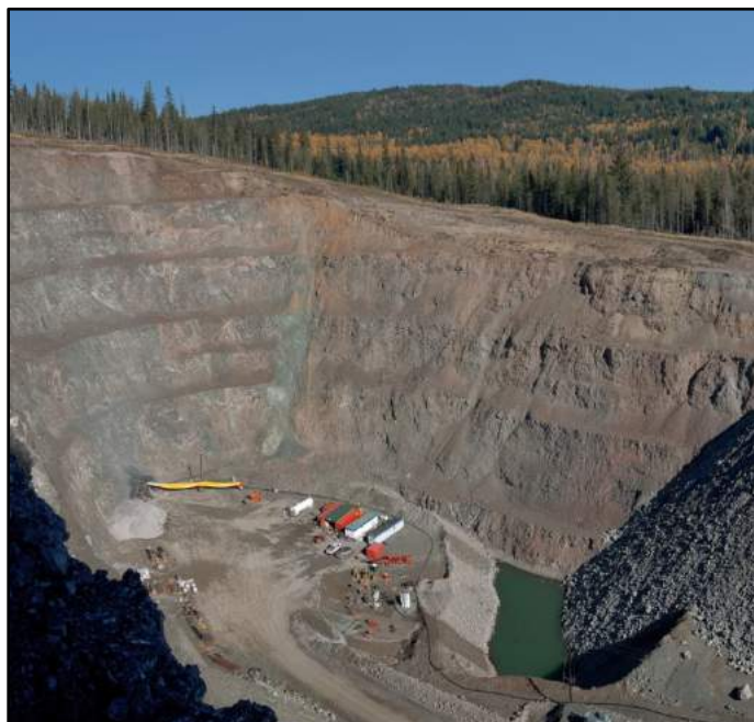
Figure 6-1 Completed Wight Pit with the Boundary UG Portal in North End
