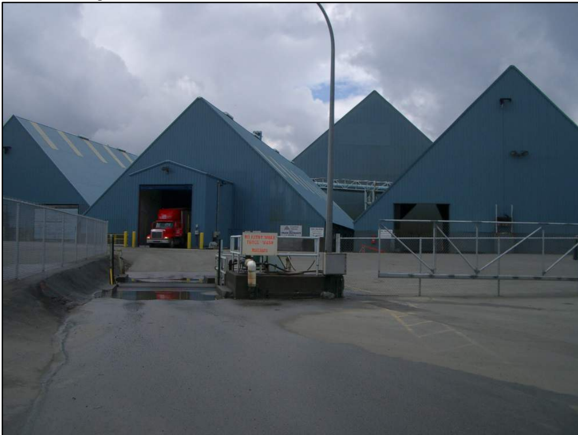
Figure 17-12 MPMC's Concentrate Shed at Vancouver Wharves
