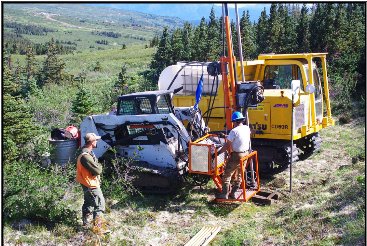
Figure 11.7 Bobcat Mounted Hydra Core Drill
