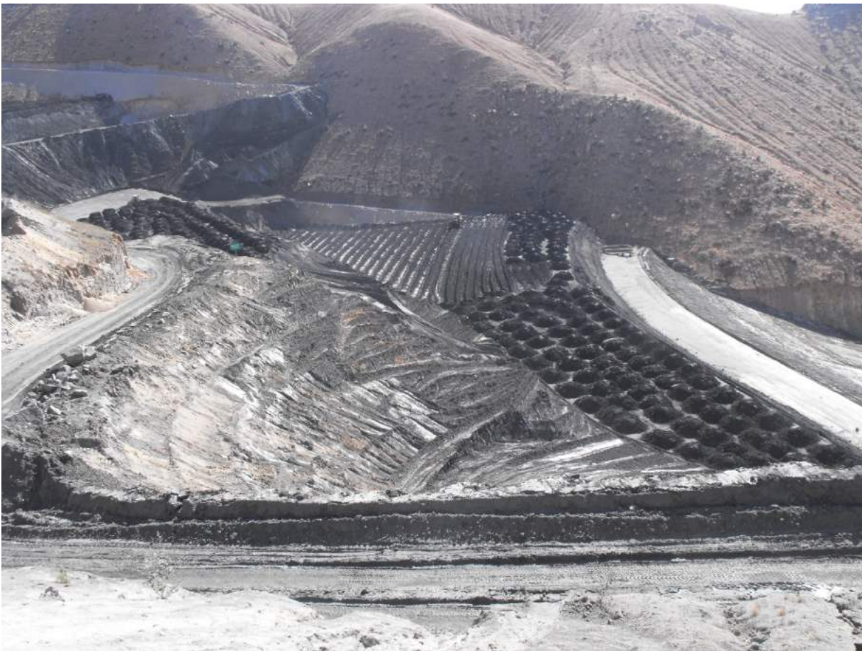
Figure 8: Placement of Filtered Tailings at Cerro Lindo Mine, Peru
