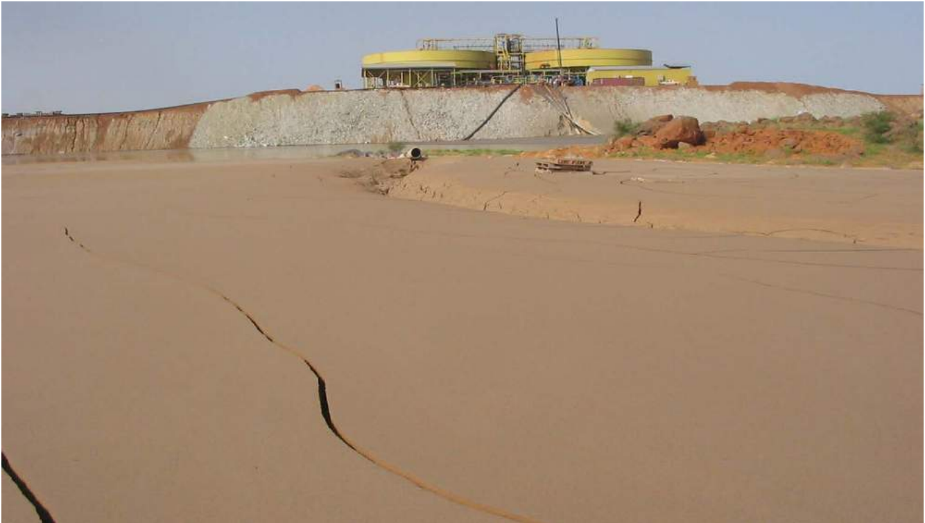
Figure 4: Thickened Tailings at the Essakane Gold Mine, Burkina Faso
