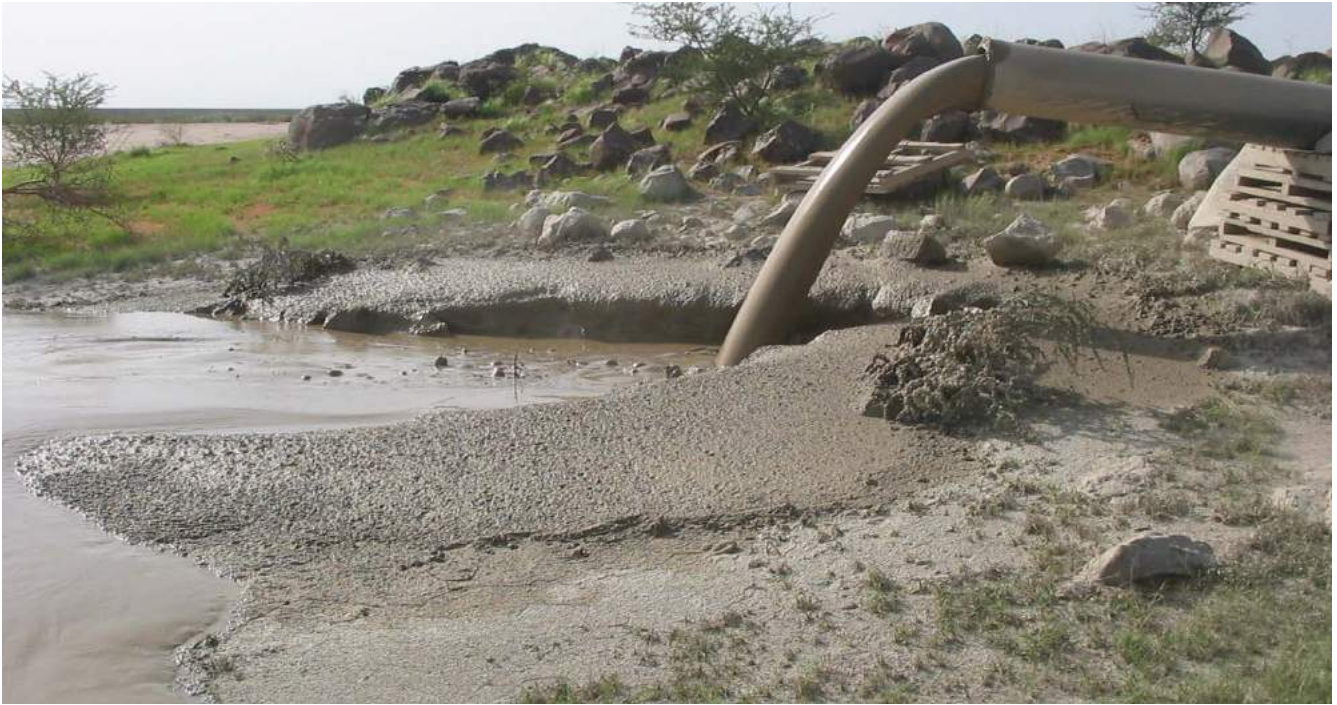
Figure 5: Discharge of Thickened Tailings (Essakane Gold Mine)
