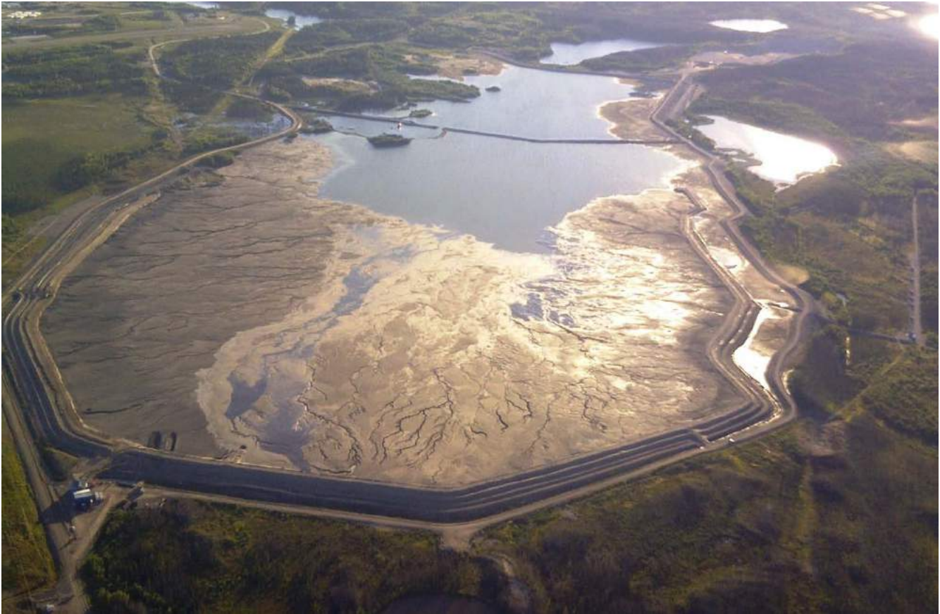
Figure 6: Thickened Tailings Storage Facility at Musselwhite Gold Mine, Canada
