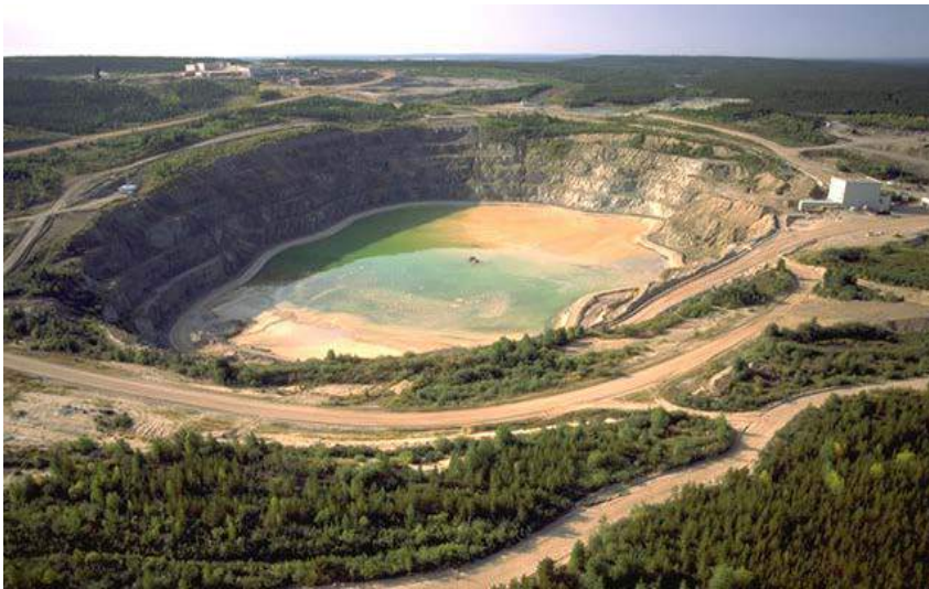
Figure 3: JEB Tailings Management Facility in Northern Saskatchewan
