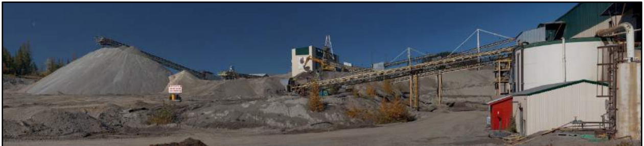
Figure 6-2 Mount Polley Crusher and Crushed Ore Stock Piles
