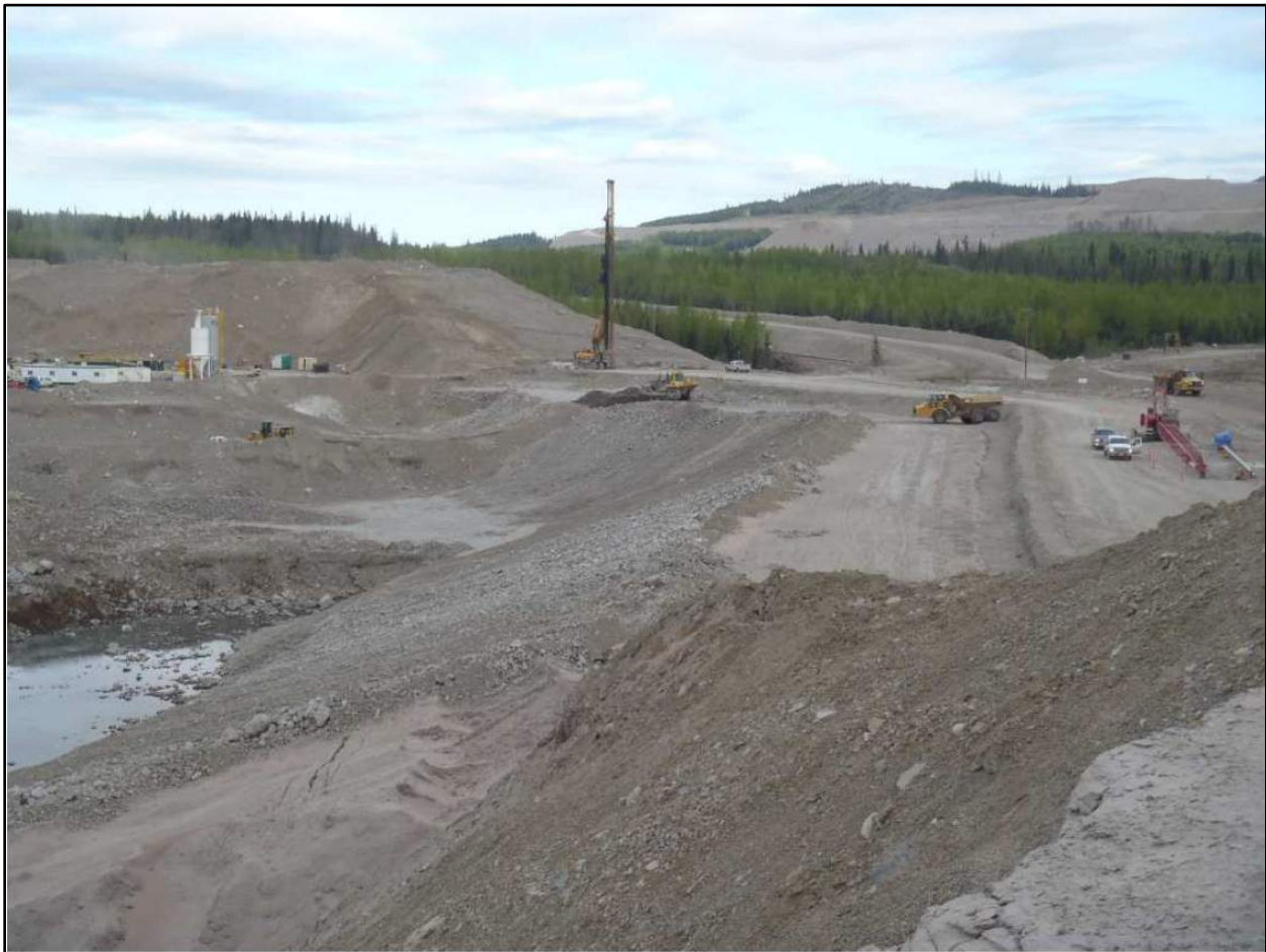
Figure 18-1 TSF Showing 950m Repair Embankment Relative to the 968.5m Embankments
