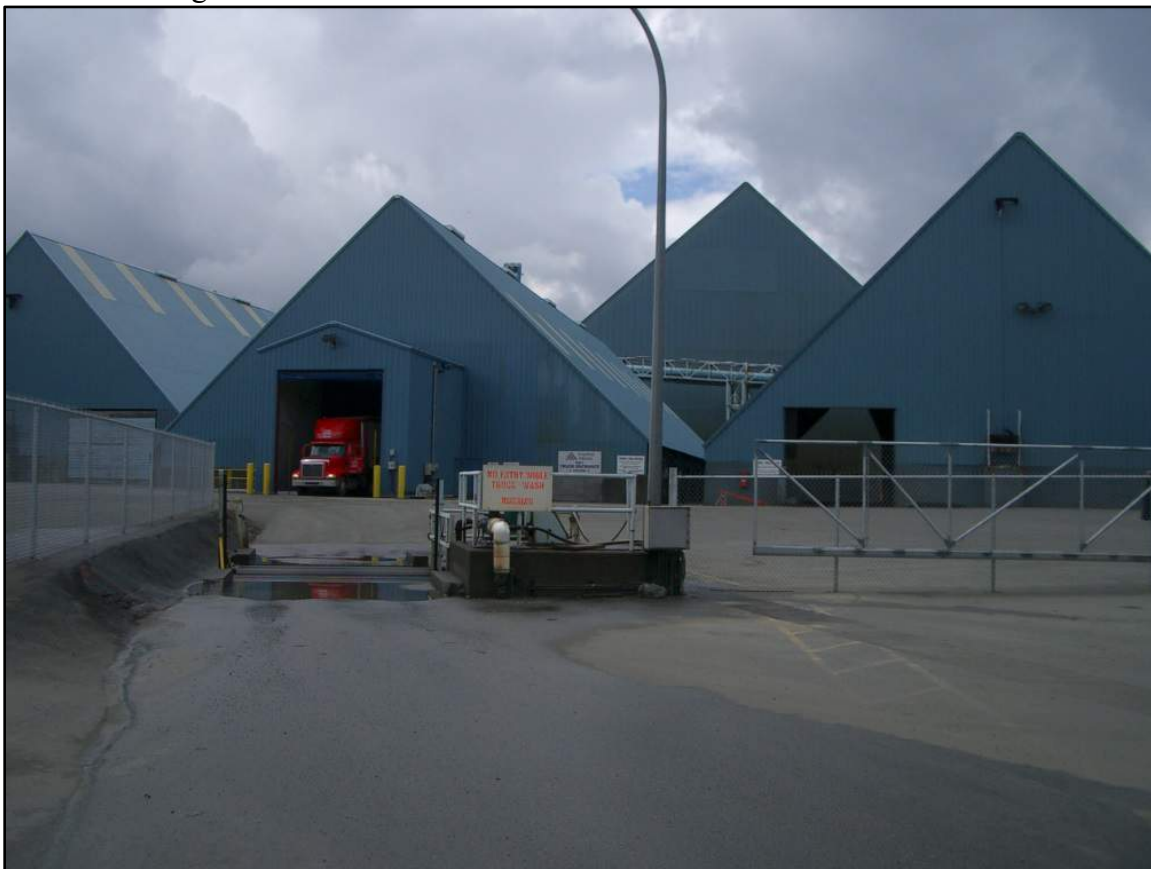
Figure 17-12 MPMC's Concentrate Shed at Vancouver Wharves
