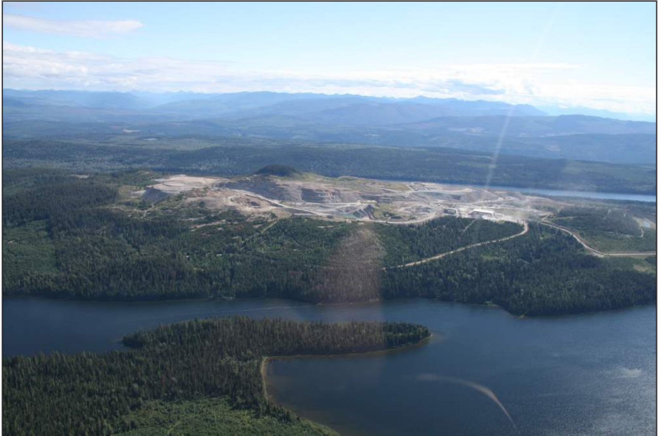
Figure 5-1 Air Photo Looking Northeast: Showing Mount Polley Mine and the Local Terrain
