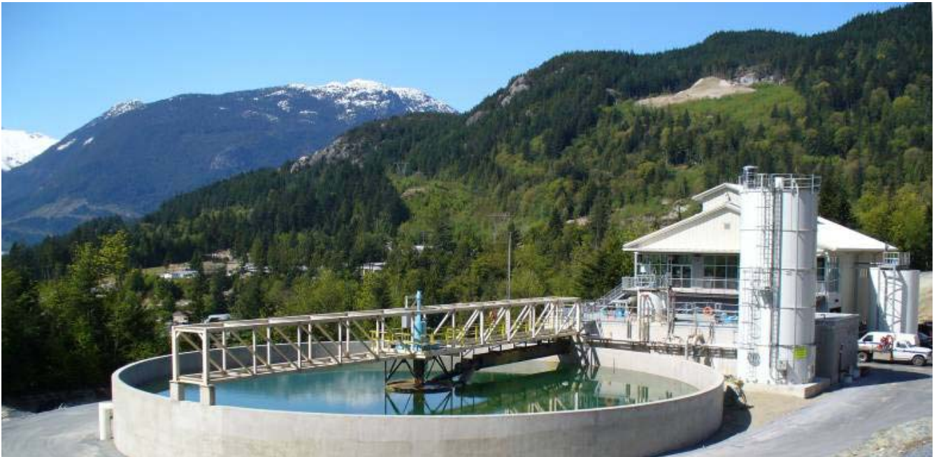
The EPCOR mine water treatment at Britannia, BC
