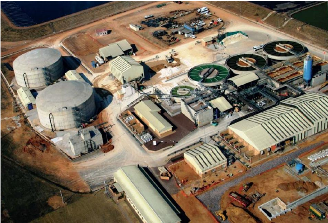
Figure 11: The eMalahleni Mine Water Reclamation Plant: South Africa (photo credit Anglo American)
