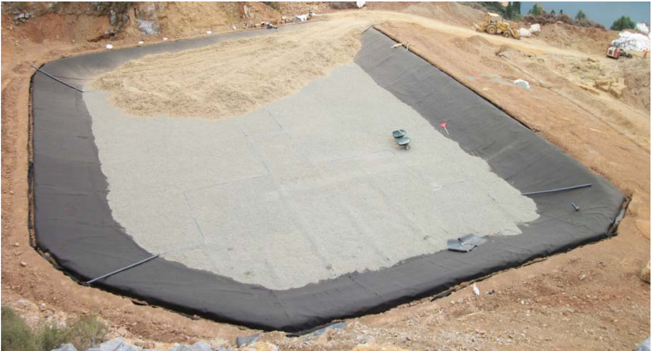
Figure 10: A passive BCR cell under construction (Golder Associates 2014)
