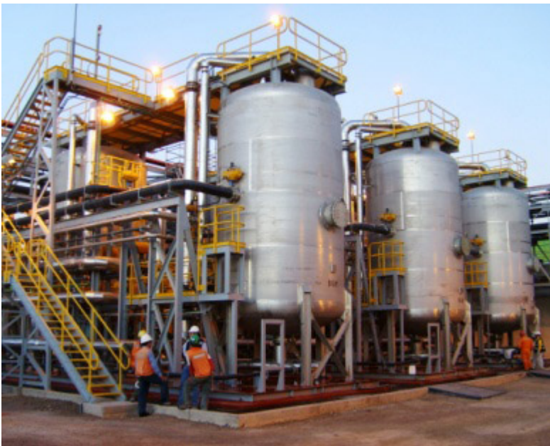
Figure 5: Dual media filter in operation at a mine (photo credit Roymec Technologies)
