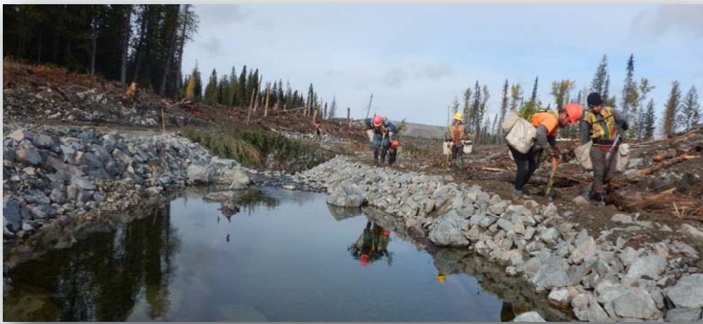
Crews planting native shrubs along Reach 2 of upper Hazeltine Creek, October 2017
