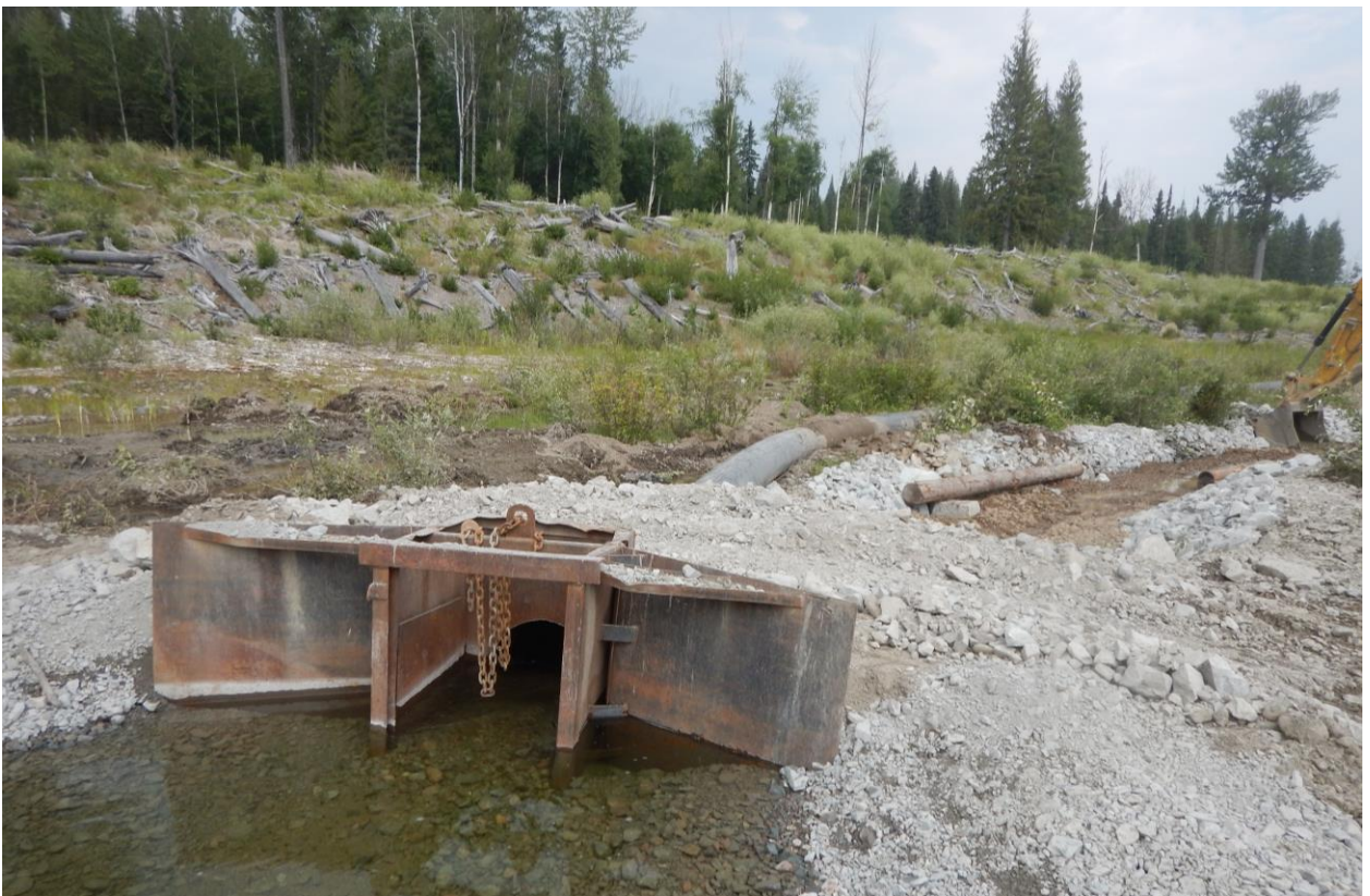
Figure 7 Water bypass pipeline used to dewater remediation worksite
