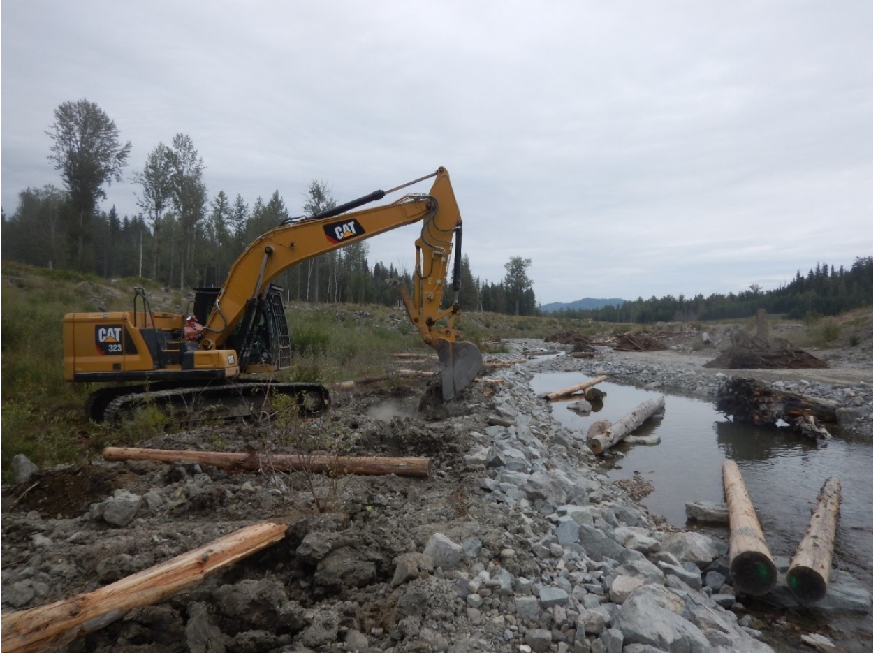
Figure 6 Surficial roughening treatment on the lower floodplains in Reach 5 of Hazeltine
