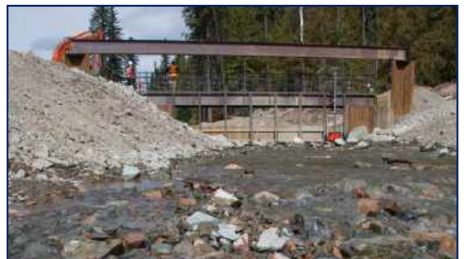
Weir structure at outlet from Polley Lake now complete
