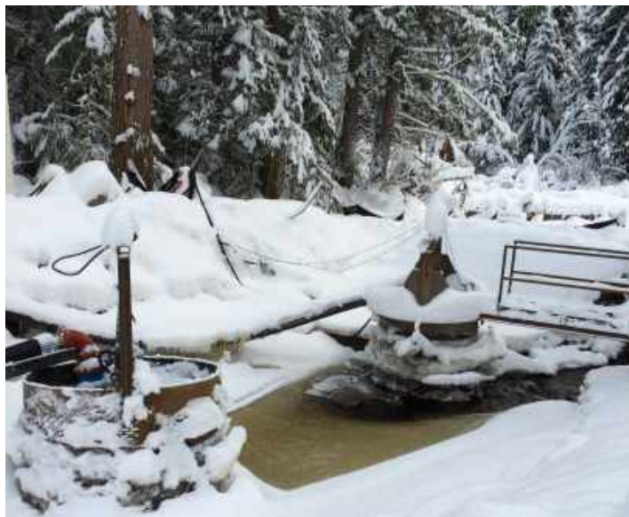
Edney Creek diversion pumps plumbed in to allow channel construction in the dry.
