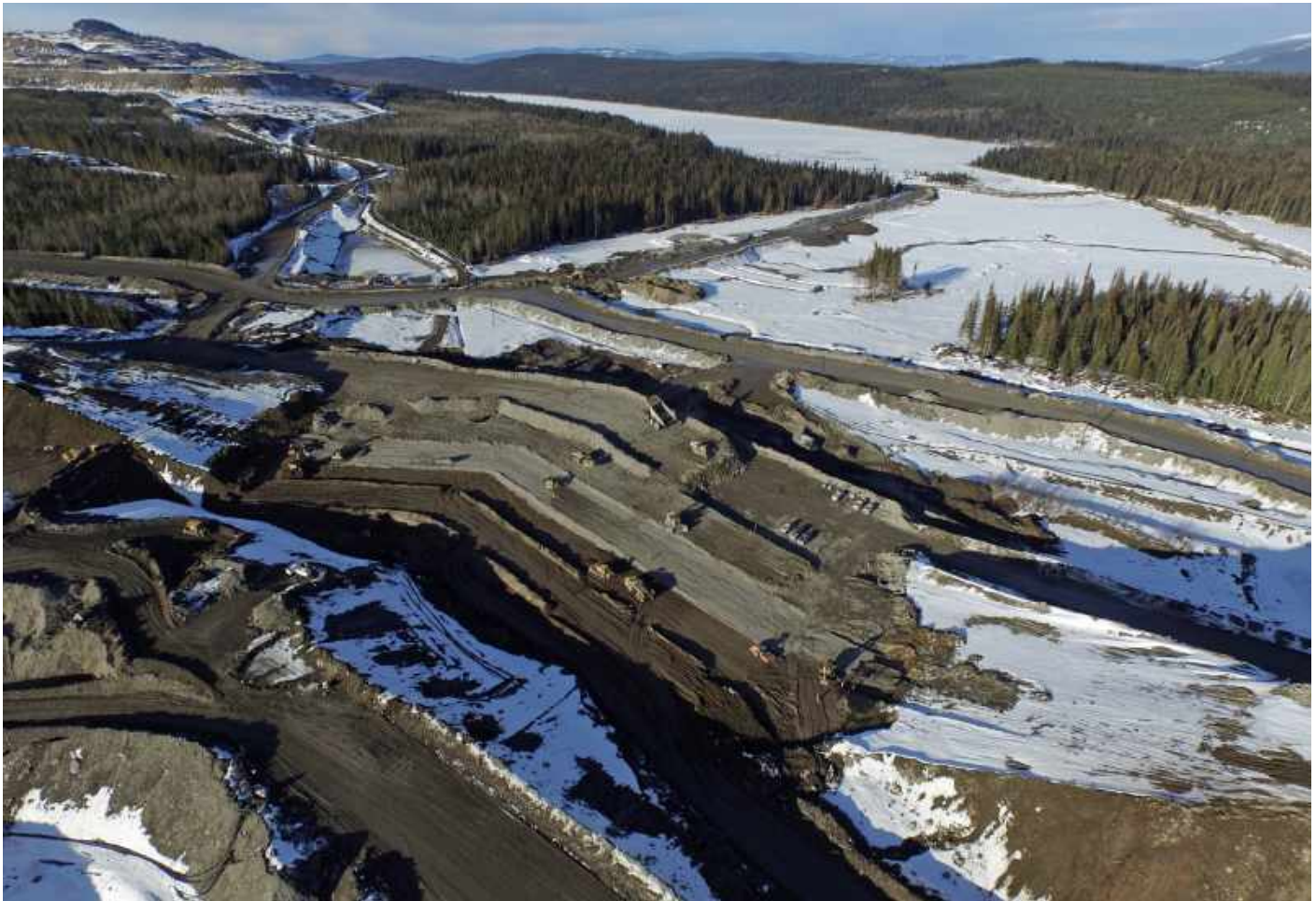
Foreground: cut-off wall for breach repair; Background: Polley Lake and Hazeltine Creek-Feb/15
