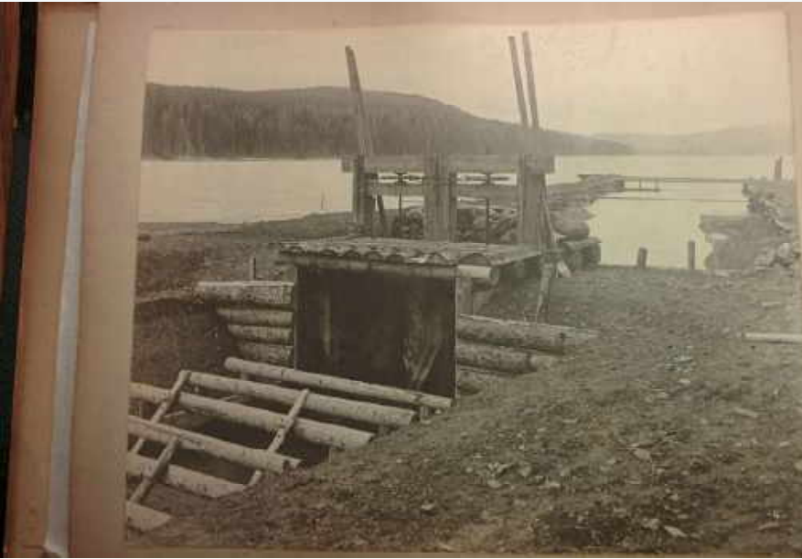
Polley Lake Outlet Structure: water works for placer mining—early 1900s. Courtesy of BC Archives.
