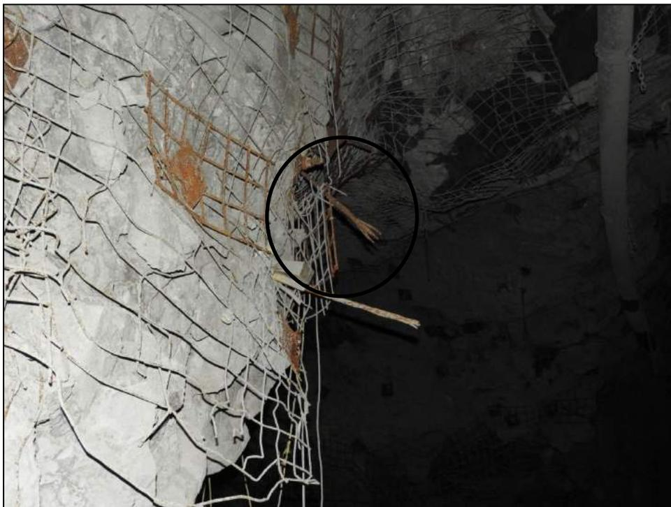
*Photograph 2: The South Wall of Block A showing a Cable Bolt that is Untwisting (Picture 2)*
