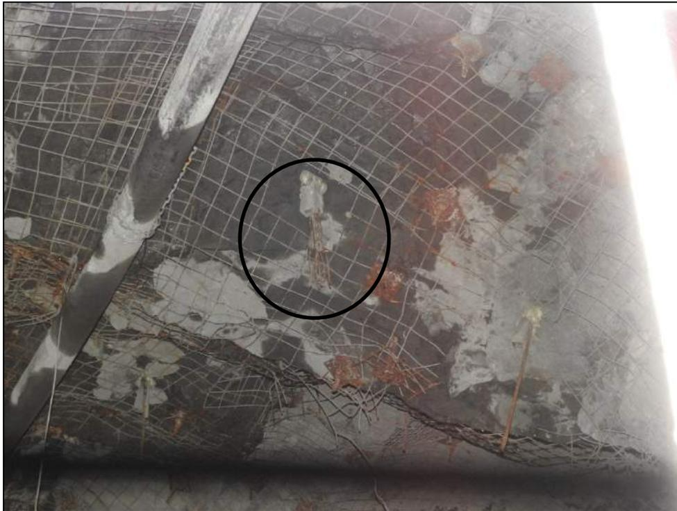
*Photograph 1: The Back of Block A Showing a Cable Bolt that is Untwisting (Picture 1)*
