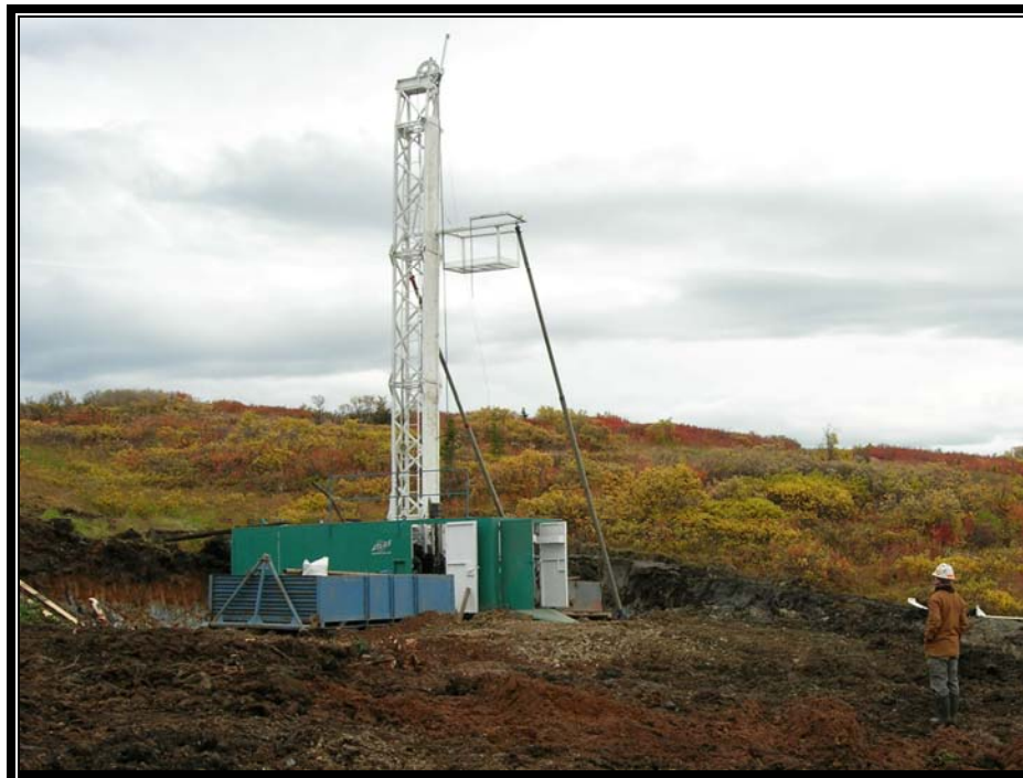
Figure 11.2 Red Chris Drilling in Progress
