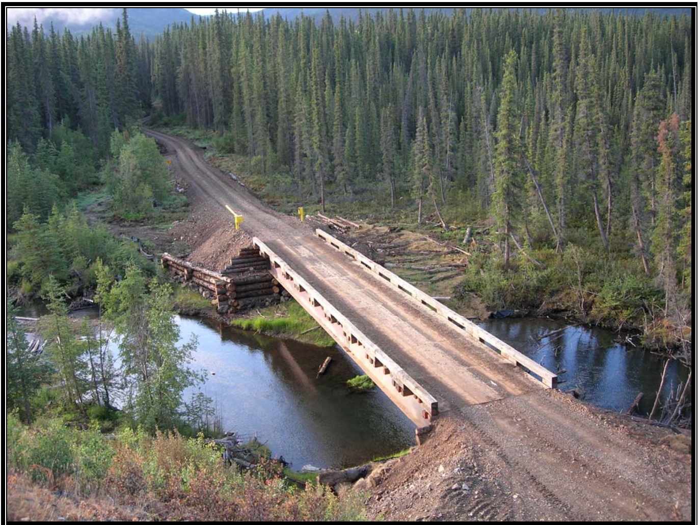
Figure 10.4 New Red Chris 17km Gravel Access Trail
