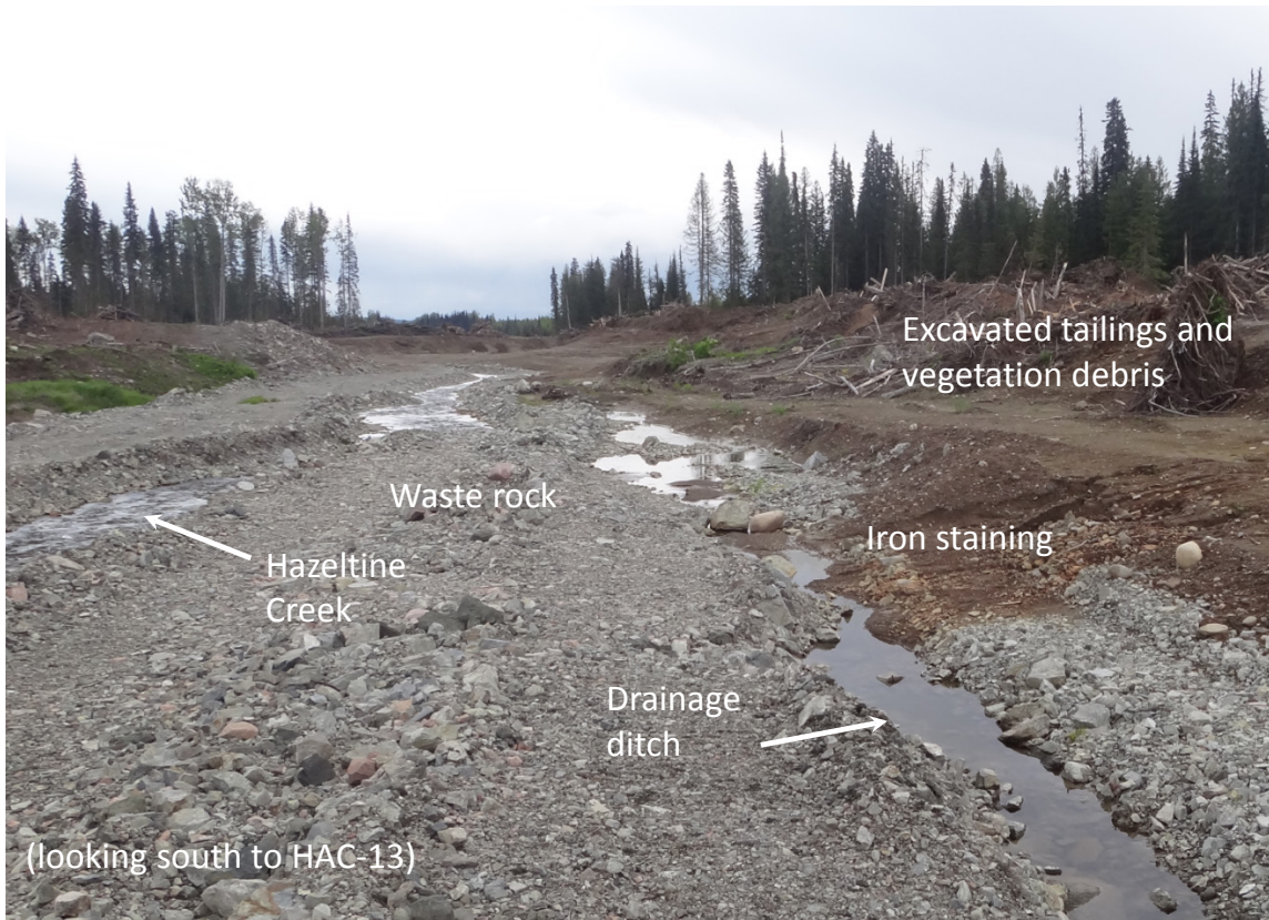
Figure 4-2: Photograph of Hazeltine Creek, drainage ditch, and excavated tailings.
