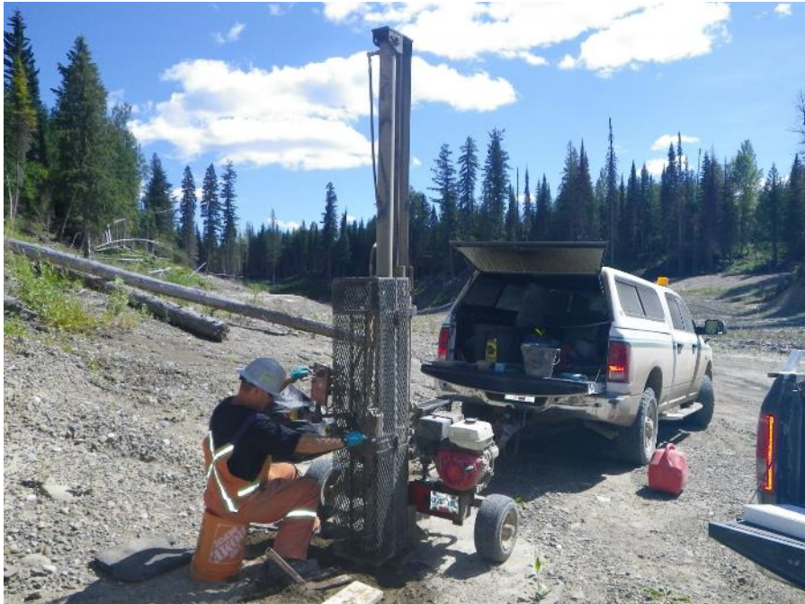
Photograph 3: Drilling MW16-06 Using the Truck-Mounted Solid Stem Auger Drill Rig
